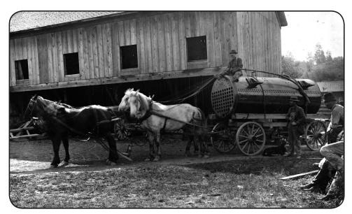
The Hanfords received the original horizontal return tube steam boiler in 1895.
