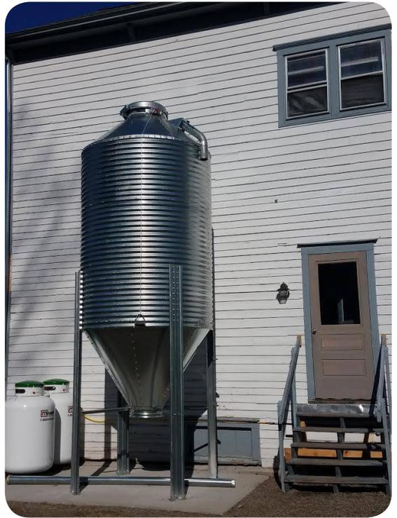
*The bulk-feed silo holds about 6 tons of wood pellets which are automatically fed into the Museum's new wood pellet boiler.*
