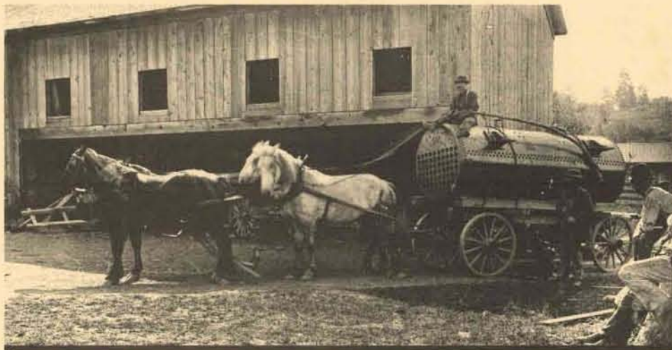
The four ton boiler arrives. Horace Hanford photographed it in front of the mill's lumber shed.
