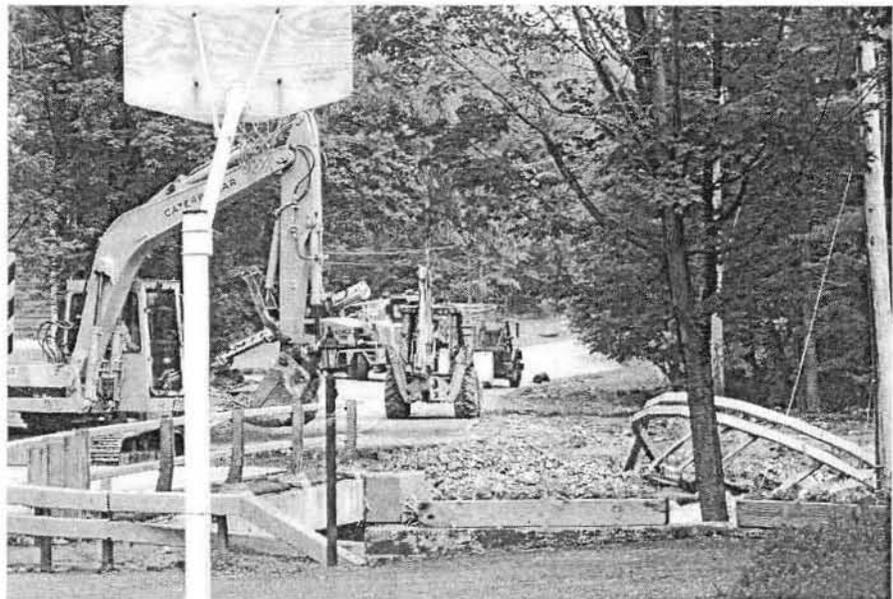
*By June 30<sup>th</sup>, road crews with machinery were already at work repairing the flood damage to the County Route 10 bridge over Kortright Creek. The bridge itself is intact, but the flood washed away part of the road in front of the bridge. Note the bent guard rail on the right.*
