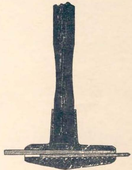
*This advertisement shows the unique type of mill pick D.J. Hanford ordered. The drawing shows how the replaceable tips were held in place.*
