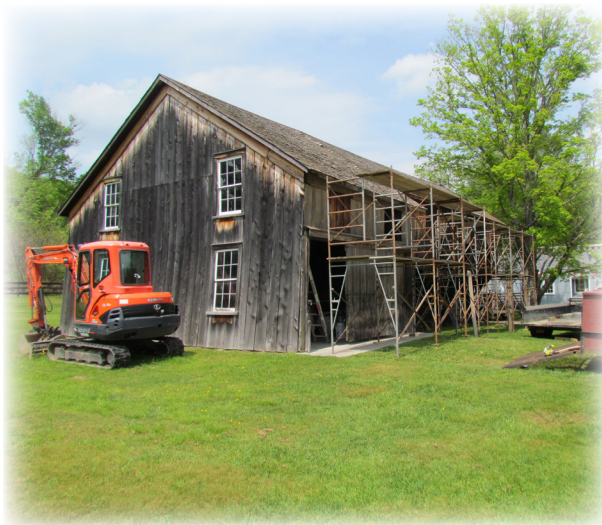
The Lumber Drying Shed is ready for its roof replacement.
