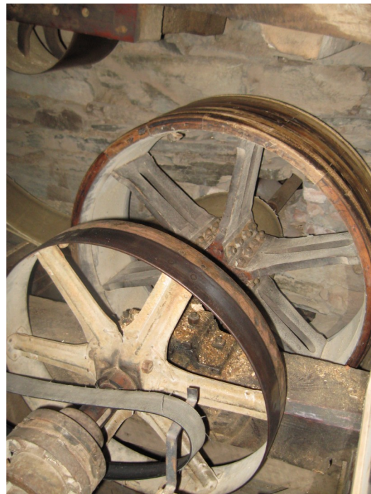
A Gilbert pulley (background next to wall) as installed on the Mill's main shaft. This 40-inch diameter pulley drives the Mill's circular saw.
