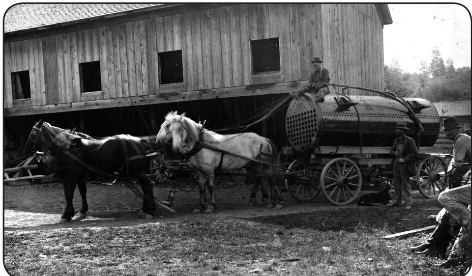
*The Hanfords received the original horizontal return tube steam boiler in 1895.*
