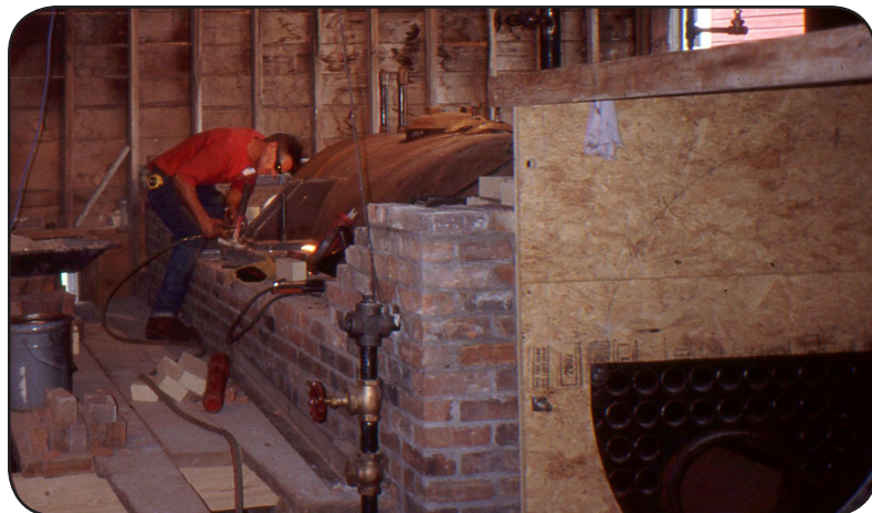
Two boilers: The Mill's original steam boiler arrived by horse-drawn wagon in 1895 (above). A nearly identical reproduction boiler was installed in 2003 and surrounded by historic bricks from the former Oneonta Roundhouse (below).
