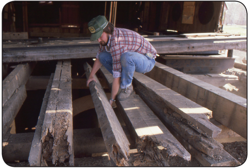
Rotted beams were removed and replaced on the Mill's main floor during restoration work in 1982.
